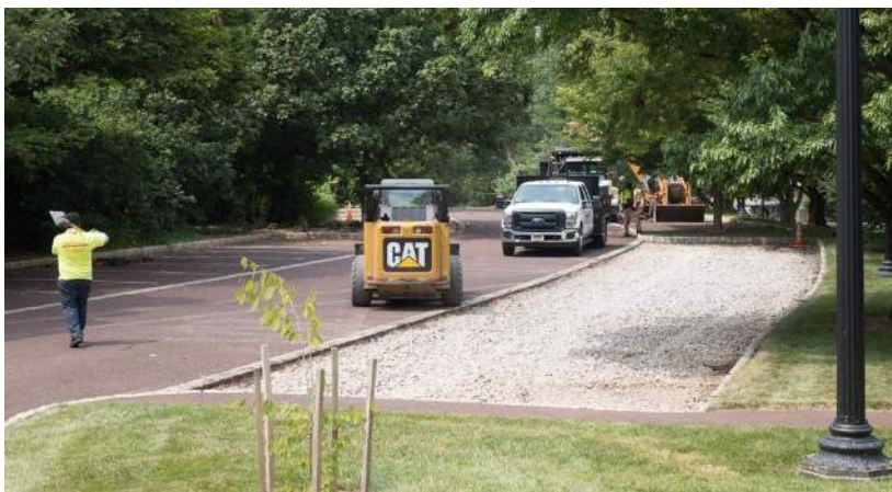
New Porous Asphalt Parking
